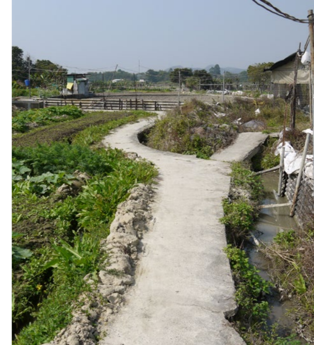
③ Concrete path
