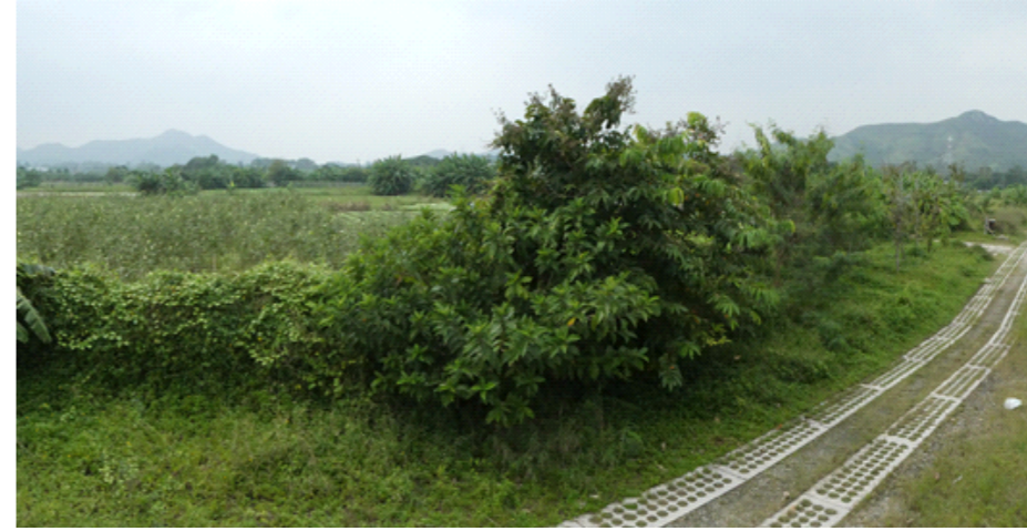
Drainage maintenance access and fences
