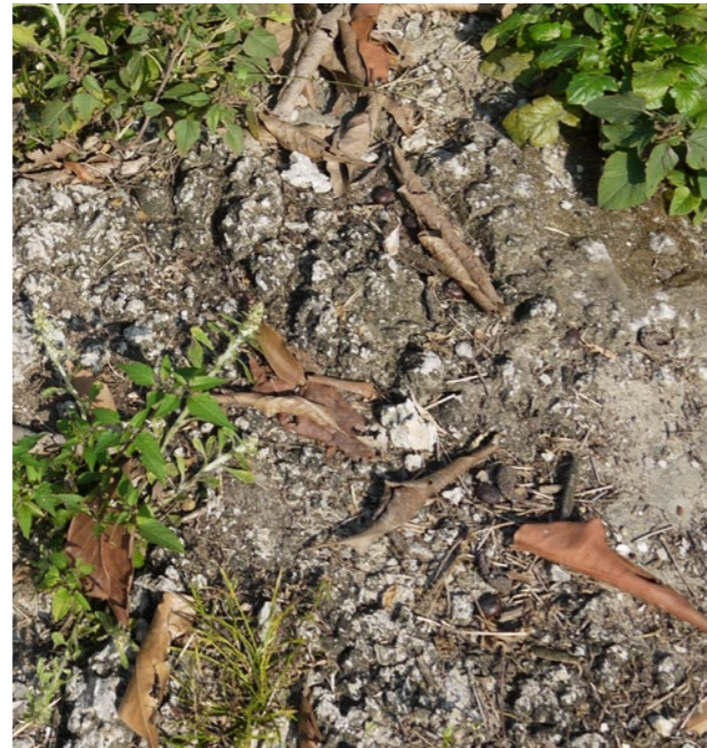
Degraded aggregate / earth path
